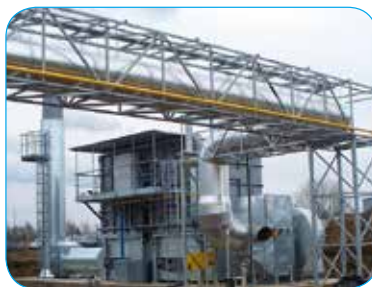
Automotive industry Air flow rate: 34000 Nm 3 /h Pollutants: ethyl acetate, xylene, MIBK
