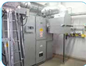
Automotive industry Air flow rate: 34000 Nm 3 /h Pollutants: ethyl acetate, xylene, MIBK
