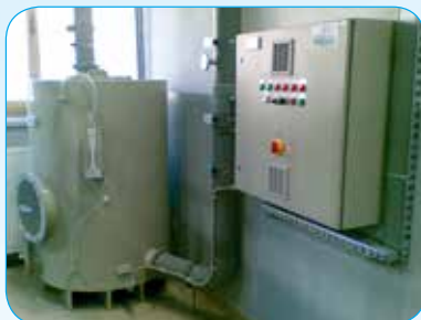
Aviation industry – core leaching autoclave system Air flow rate: 500 m 3 /h Pollutants: NaOH fumes
