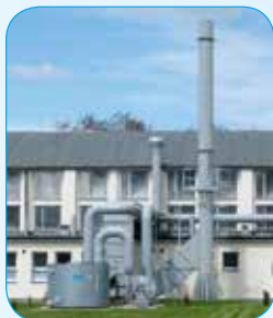
Aviation industry – surface preparation Air flow rate: 8000 m 3 /h Pollutants: acetone, isopropanol
