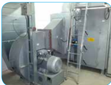
Production of abrasives Air flow rate: 23000 Nm 3 /h Pollutants: ethanol, methanol, methoxypropanol
