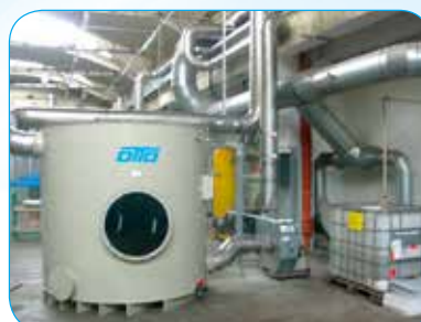
Aviation industry – blade etching Air flow rate: 2 500 m 3 /h Pollutants: VOC, Ranclene fumes, Trisol fumes
