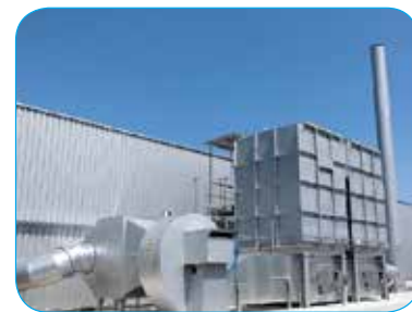
Automotive industry Air flow rate: 27000 Nm 3 /h Pollutants: xylene, MIBK, ethyl benzene, ethyl acetate, acetone, ethyl acetate, MEK
