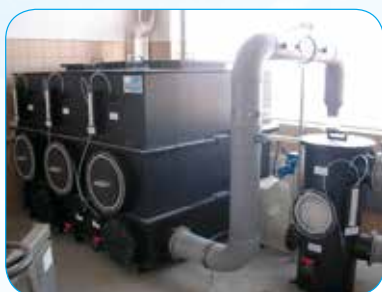
3-stage adsorber – municipal sewage treatment plant - pre-treatment area Air flow rate: 1 000 m 3 /h Pollutants: Odours, hydrogen sulphide, ammonia
