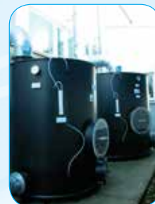
Aviation industry – Plating shop Air flow rate: 7000 m 3 /h Pollutants: VOC and paraffin fumes
